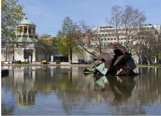
Parts of the roof of the Opera house were blown down.
